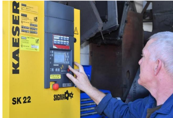
Caption: Kaeser recommended and subsequently installed an Aircenter SK 22 to replace the ageing compressor at Trevor French Radiators.
