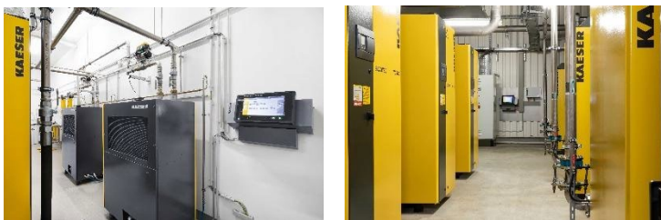
Caption: The latest generation of compressed air management systems, such as the Sigma Air Manager 4.0, now provide a range of enhanced benefits with a view to achieving optimisation of the entire system.
