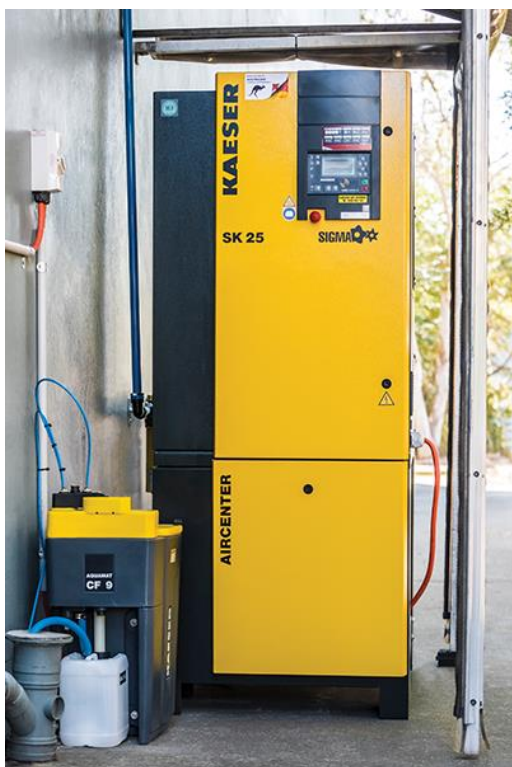
Caption: Bright chose to replace an ageing compressor with a new Kaeser Aircenter 25
