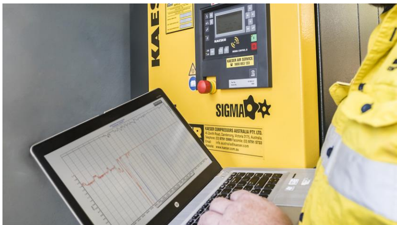
Caption: Kaeser was invited to perform a complete Air Demand Analysis (ADA) on the existing compressed air system
