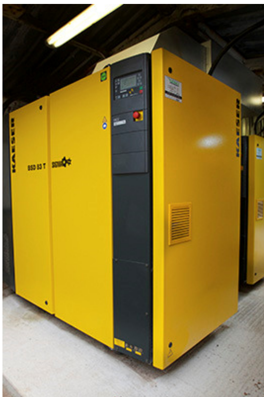
Caption: A Kaeser ASD 50 T and a BSD 83 T rotary screw compressor, both with integrated refrigeration dryers installed at Katere Coatings
