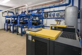
Caption: Two Kaeser SX 3 T series rotary screw compressors with integrated refrigeration dryers, complete with air treatment package and air receiver installed at Bannister Downs Dairy Farm.
