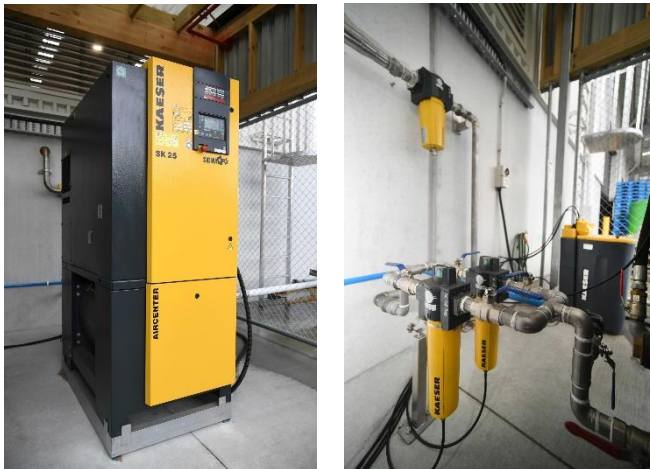
Caption: The Kaeser Aircenter all-in-one compressed air station, complete with filtration at Suntory Coffee.
