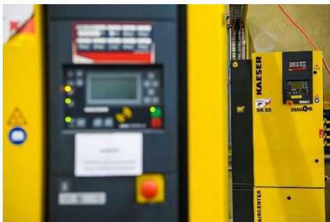
Caption: The Kaeser Aircenter SK25 and two Kaeser ASK 34 T's also in operation at Victor Footwear to meet the facilities compressed air requirements.
