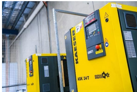
Caption: The Kaeser Aircenter SK25 and two Kaeser ASK 34 T's also in operation at Victor Footwear to meet the facilities compressed air requirements.
