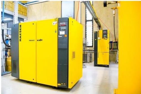
Caption: The Kaeser BSD 65 T selected to meet the additional compressed air requirements of the new direct injection moulding machine at Victor Footwear.
