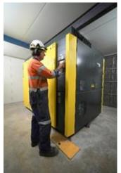
Caption: The Kaeser DSDX 305 series rotary screw compressor at Golden Bay Cement's manufacturing plant in Whangarei, New Zealand.
