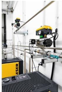
**Caption:** The DHS 4.0 air-main charging system from Kaeser protects the compressed air treatment components, and helps ensure reliable compressed air quality - even following a complete shutdown.
