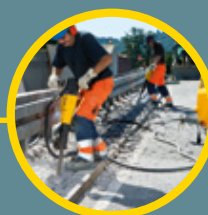
2 x 17 kg Demolition hammers
