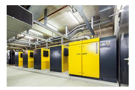
The innovative and energy-efficient FBS series screw blowers from Kaeser provide an effective and dependable supply of low pressure quality compressed air.
