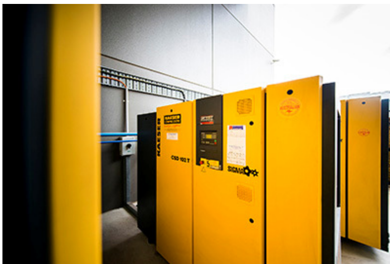
Caption: As part of the development of its power and distribution transformer capability WTC chose to invest in six Kaeser CSD series rotary screw compressors.
