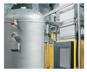
Pressure vessels - or air receivers - are an integral part of a compressed air system. Most compressed air users will have at least two pressure vessels within their compressed air system; the external air receiver and the internal air receiver - like an oil separator - which can be found within, for example, a screw compressor.
