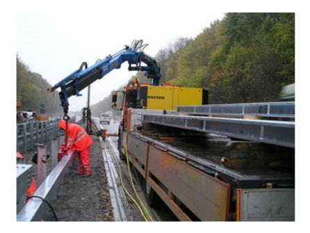
The compact M57 Utility from Kaeser combines the advantages of a modern stationary screw compressor with the location flexibility of a portable compressor
