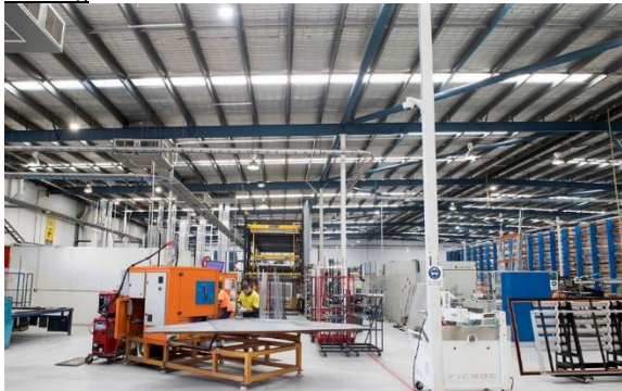
015_Image 4_compressed air application at Prowler Proof.jpg
