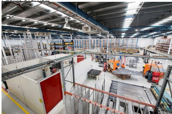
015_Image 3_Prowler Proof facility.jpg
